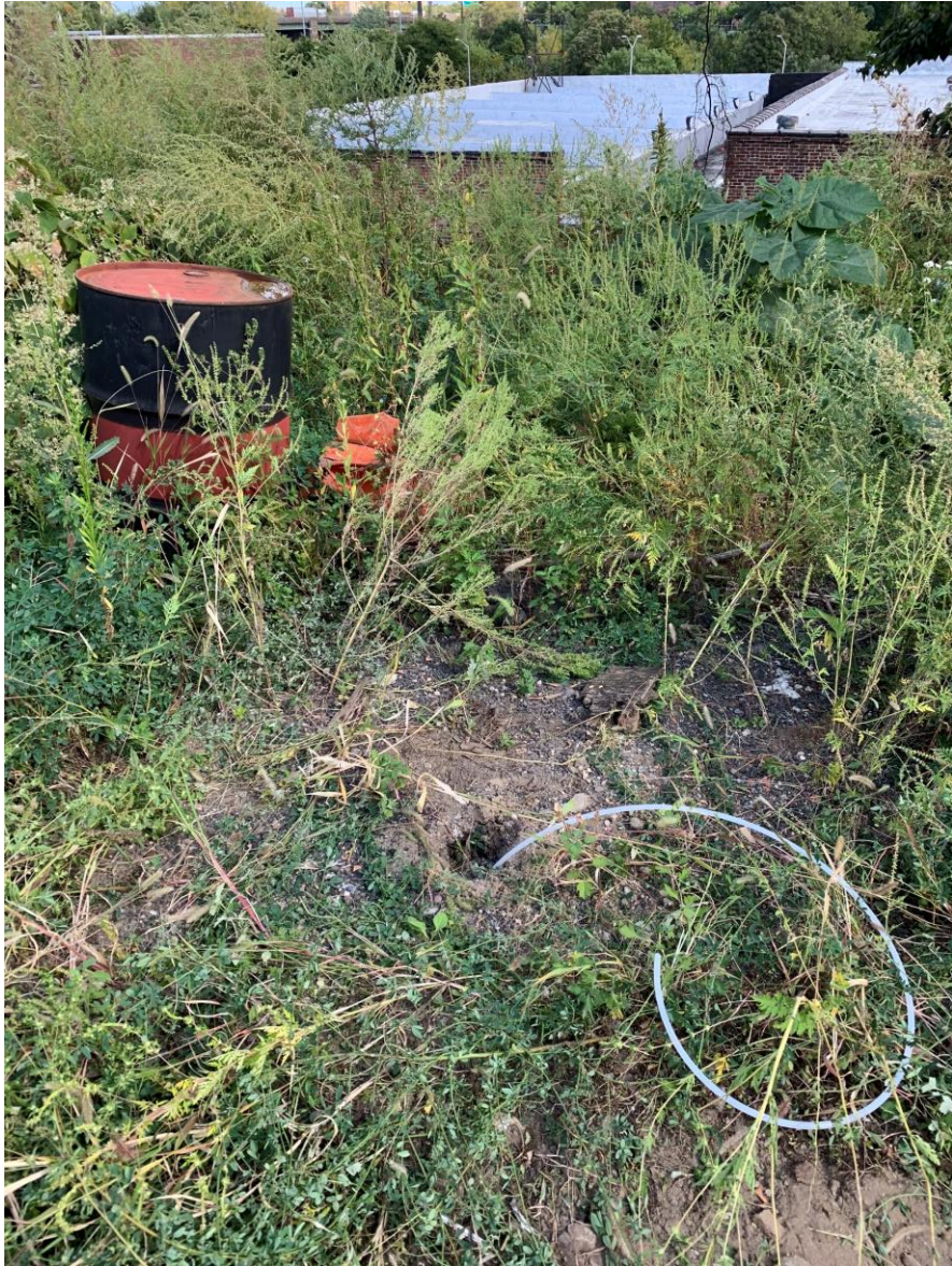
Soil vapor probe installation in process
