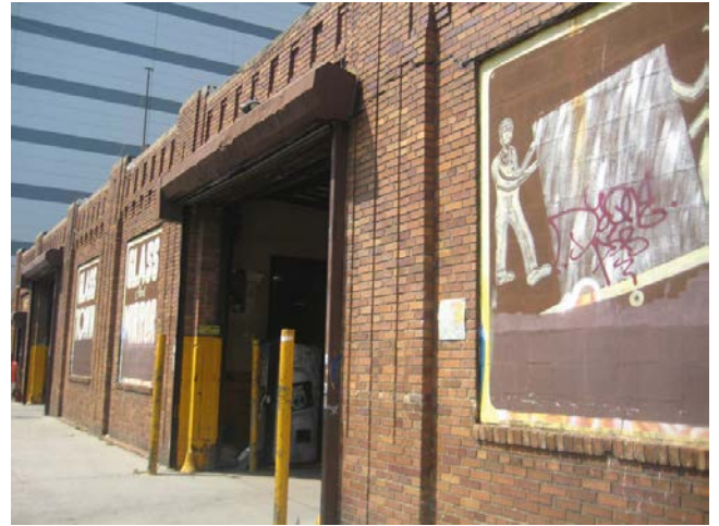
18. View of the adjacent site to the south along Gerard Avenue.
