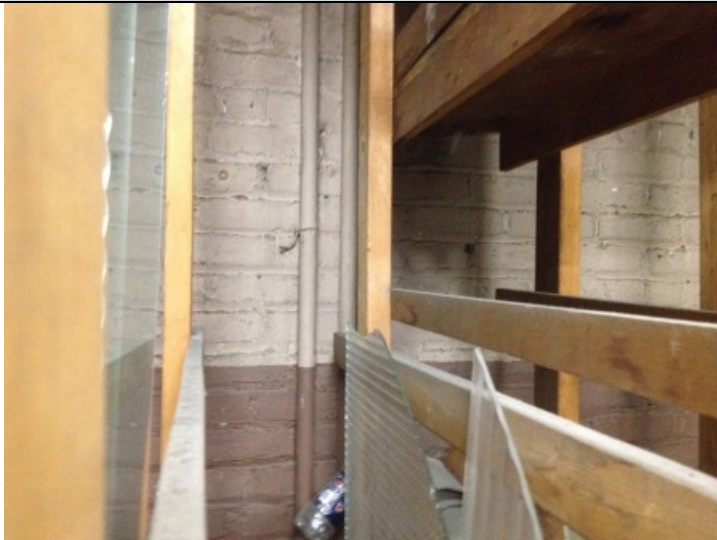
PHOTO 11: Looking at two gas tank vent lines that run up along the front wall of the building.
