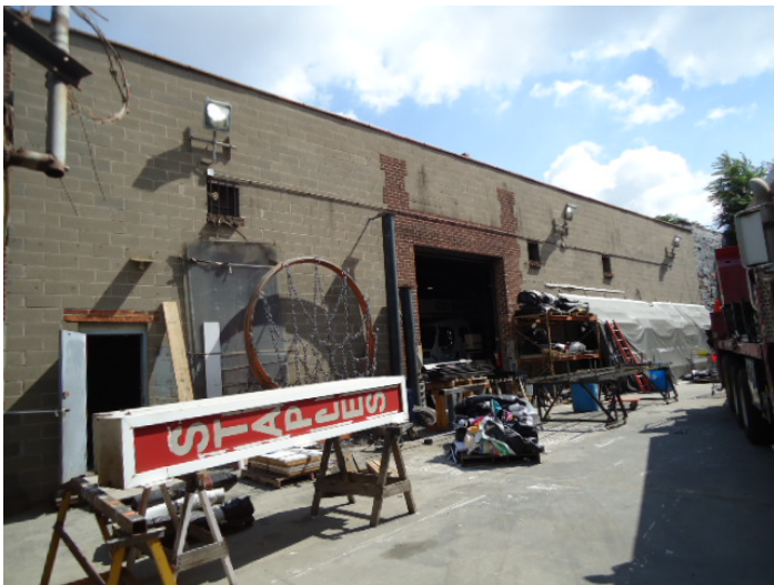
3. Southern elevation of building, facing northeast
