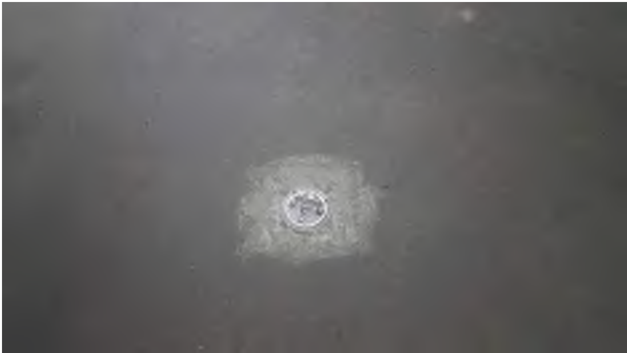
Photograph 16: One of four monitoring wells observed in basement.
