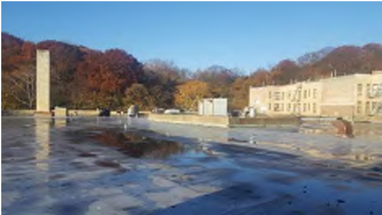
Photograph 2: Rooftop of Subject Property facing west.
