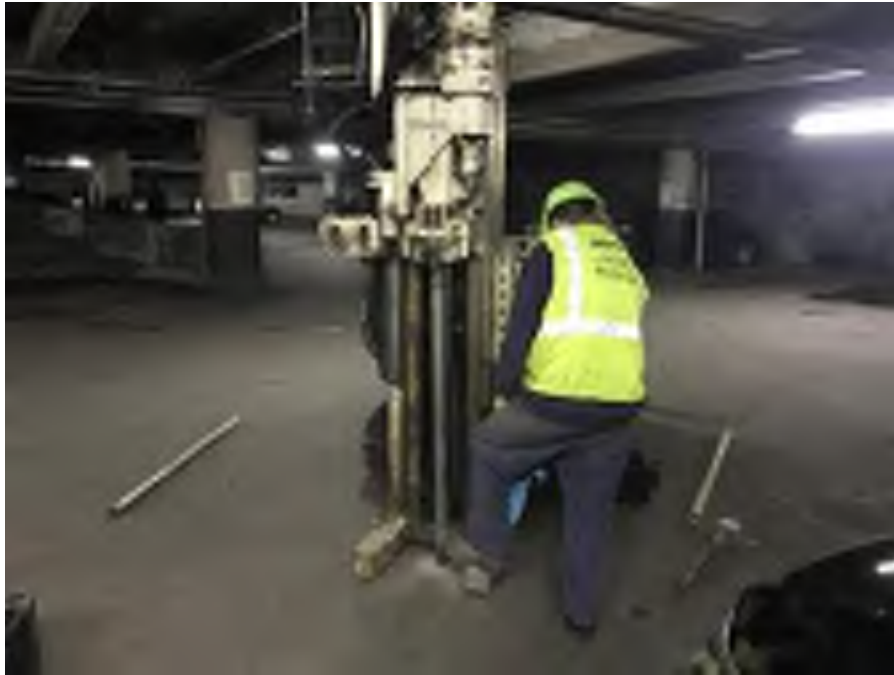
Photo 3: View of Eastern advancing a soil boring. (facing northeast)
