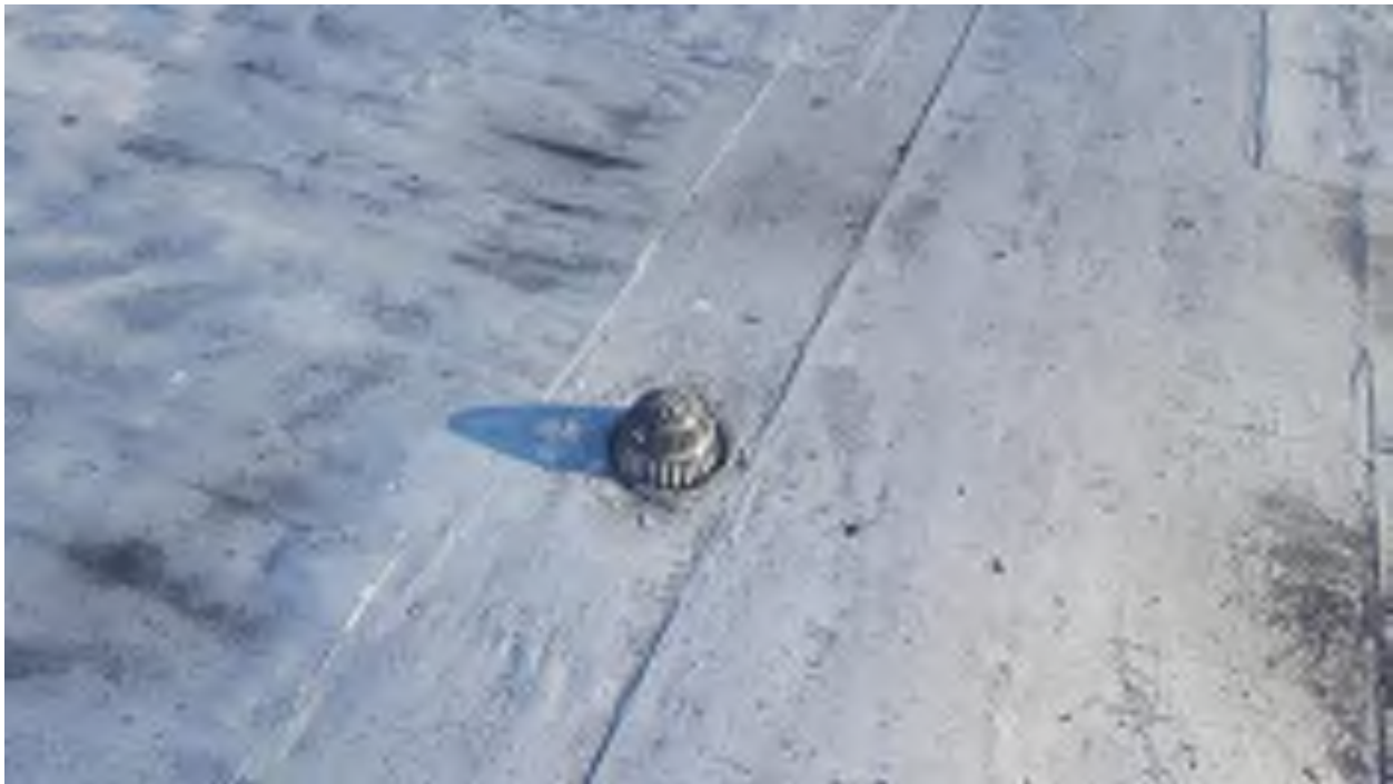
Photograph 4: Typical rooftop drain. No staining observed.
