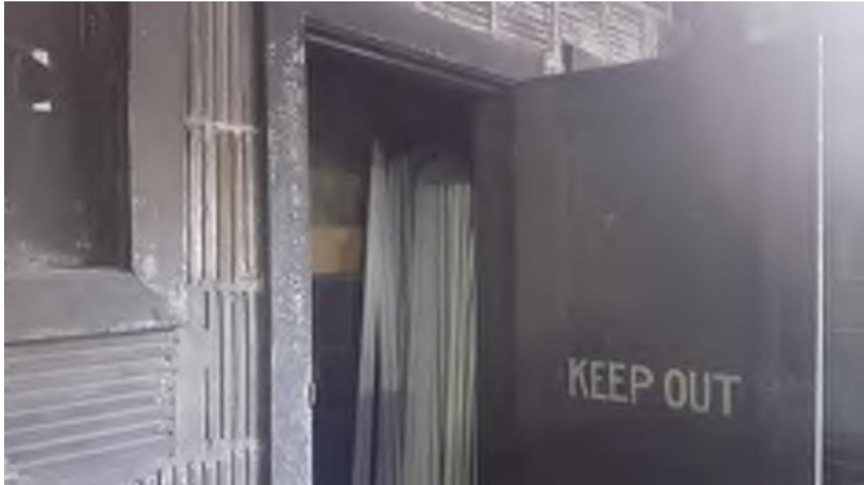
Photograph 27: Fluorescent light tubes stored in closets throughout Subject Property.
