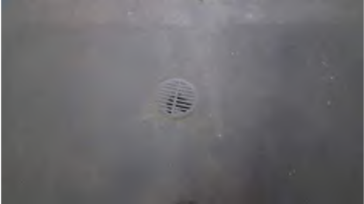
Photograph 25: Typical interior floor drain in basement.
