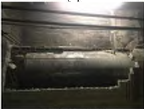
Partially exposed AST
