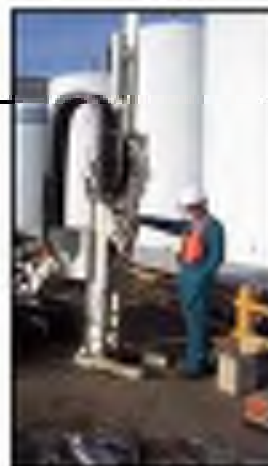
Figure 1. On Site Direct Push Injection
