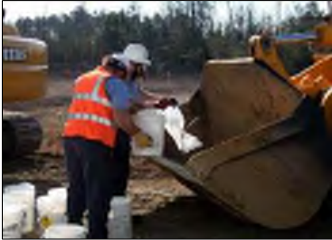
Figure 2: Application of RegenOx with a Front End Loader.
