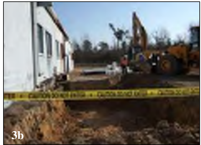
Figure 2: Application of RegenOx with a Front End Loader.
