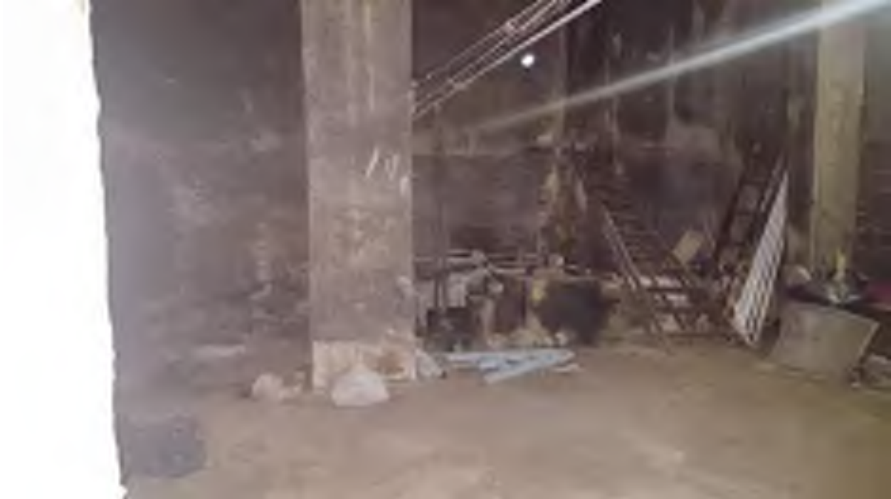
Photograph 21: Former tank room in sub-cellar.
