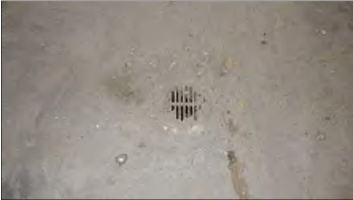
Photograph 9: View of floor drain on second floor.
