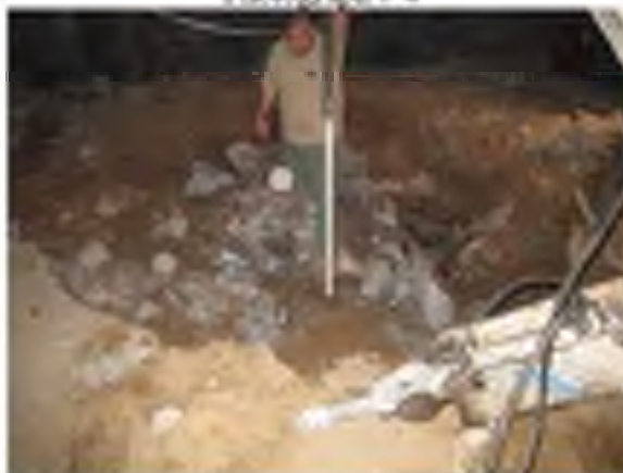
Pumping out USTs
