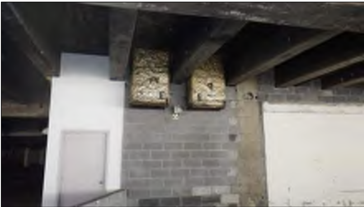
Photograph 10: View inactive ceiling-mounted heating unit on second floor.
