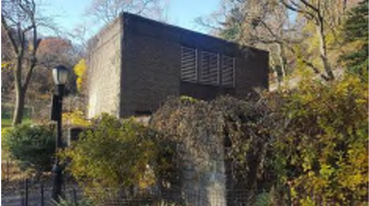
Photograph 31: Subway entrance and vent structure about 300 feet northwest of the Subject Property.
