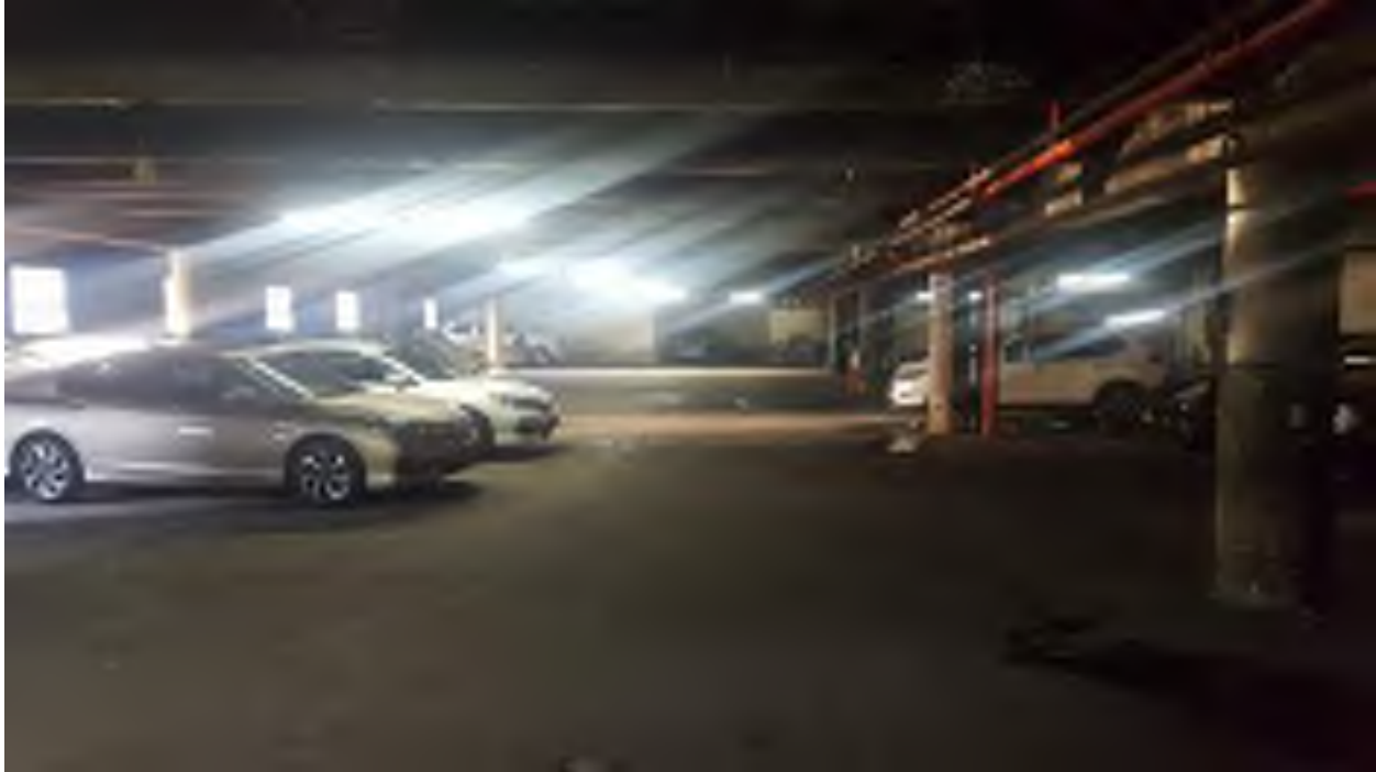
Photograph 5: Typical vehicle storage on first and second floor of parking garage (southern portion of Subject Property).
