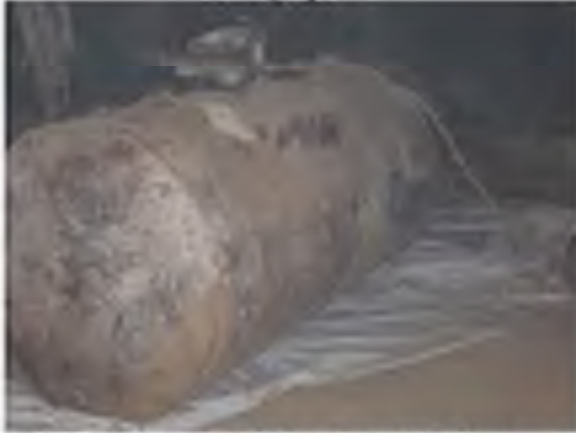
USTs removed and placed on poly sheeting.
