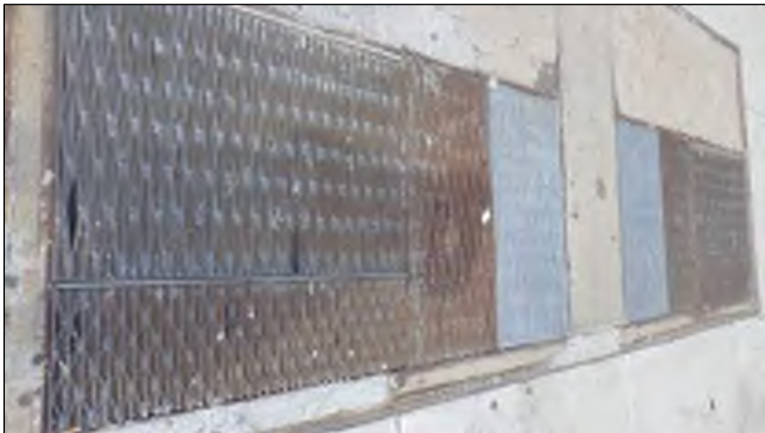
Photograph 2: View of transformer vault on Sherman Avenue.
