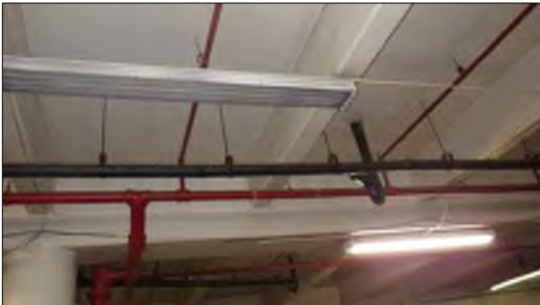
Photograph 8: View of exposed pipes and fluorescent lights on the first floor.
