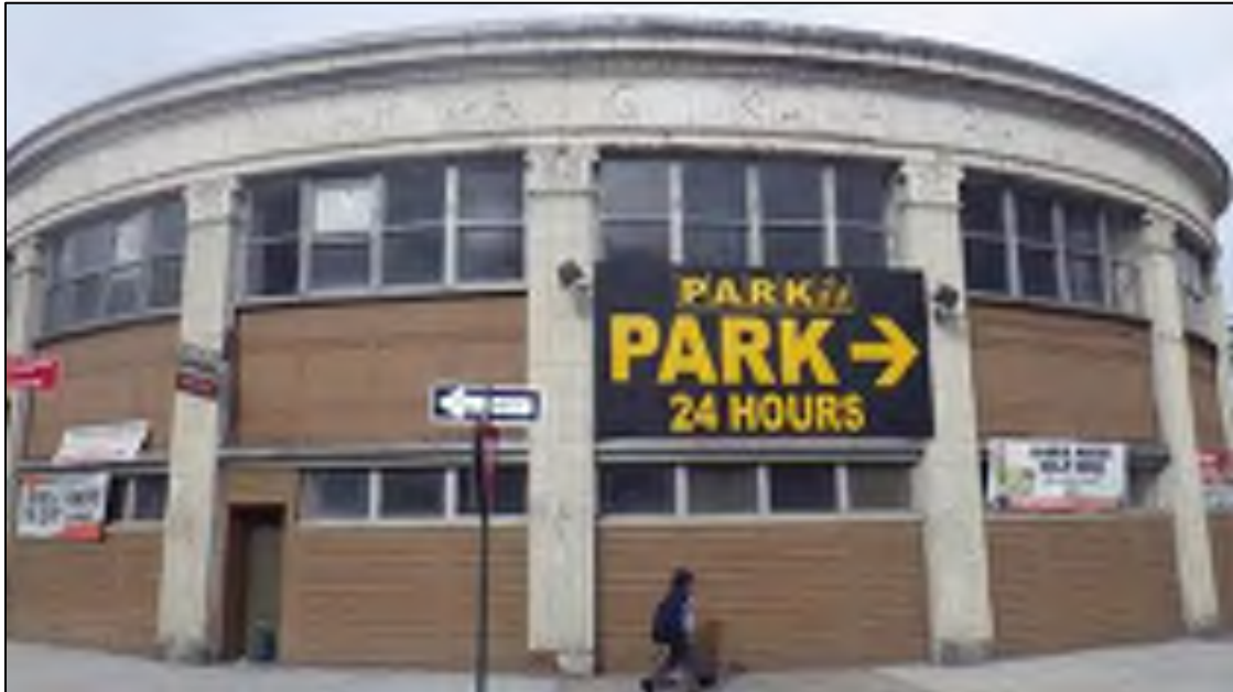
Photograph 1: View of Subject Property building from south.
