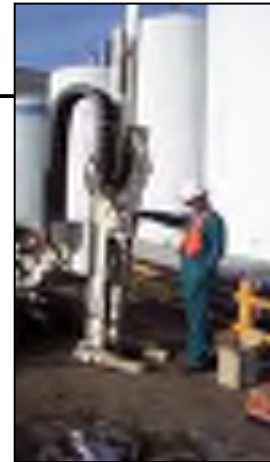
Figure 1. On-Site Direct Push Injection
