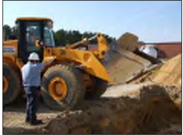
Figure 2: Application of RegenOx with a Front End Loader.
