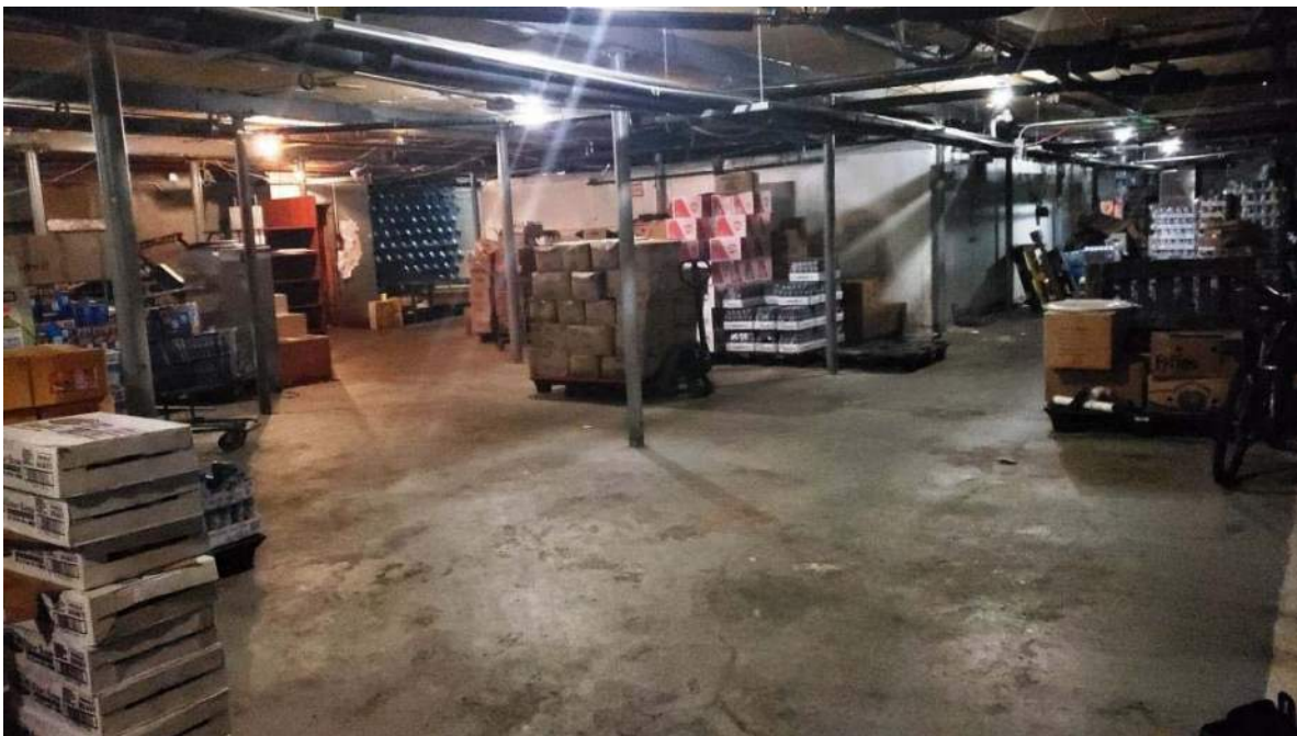
Photograph 6: General view of the grocery store basement looking south from the stairs.
