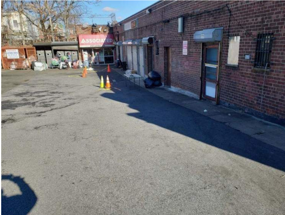
Photograph 5: Rear of the Site building. Safety cones mark the location of Soil Boring B2, which was placed adjacent to a storm grate.
